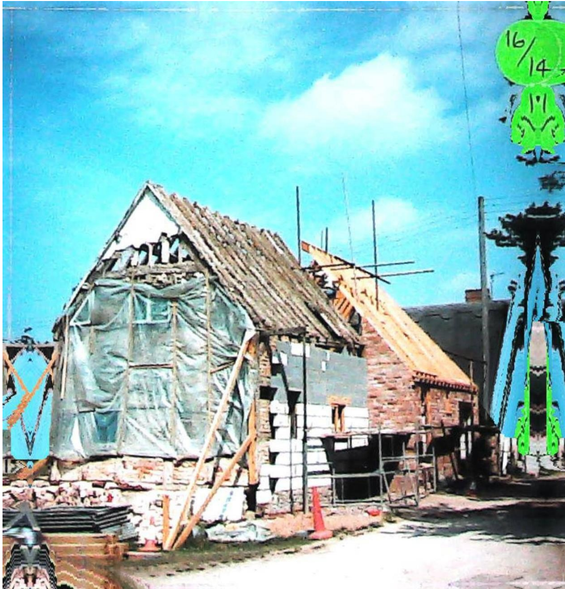
A timber-framed cottage stripped to its frame and props during restoration, probably in the 1980s. The archive links this run of photographs (16/14–17) to the restoration of Glebe Cottage by C. Padbury & Son, whose van appears in 16/17.
