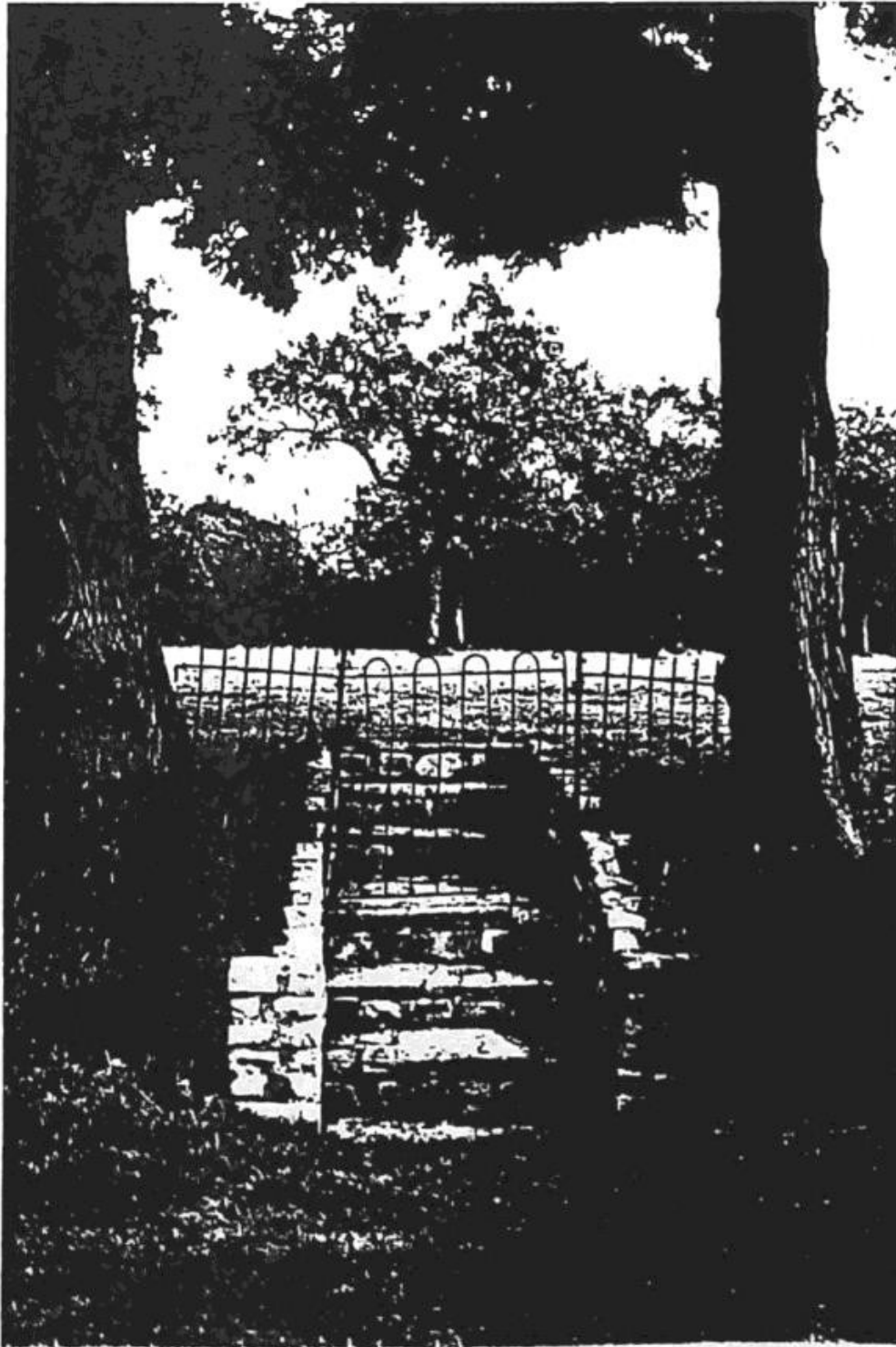
The old orchard opposite Manor Farm "with its unusual flight of stone steps and ornamental entrance gate" (15/08, fig. 25). The steps and gate are one of the seven features listed in Appendix C as "important to the Conservation Area".
