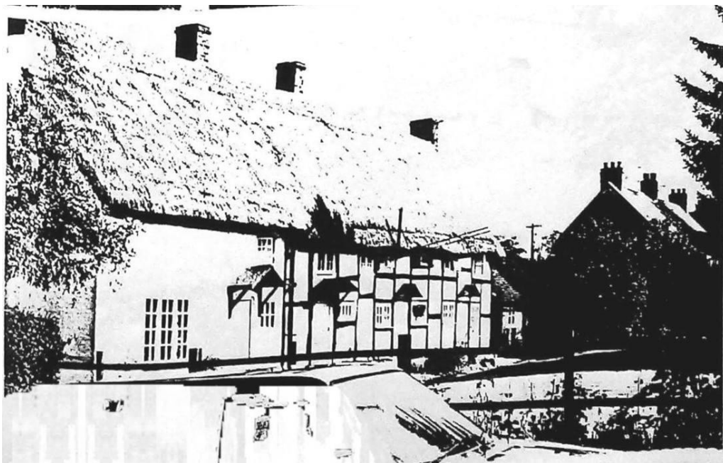
Nos 1 to 4 Sykes's Cottages, Chapel Street, "range of four two storey cottages set at right angles to road, the northernmost cottage having been rebuilt in colour washed brick" (15/08, fig. 52 and ref 22).
