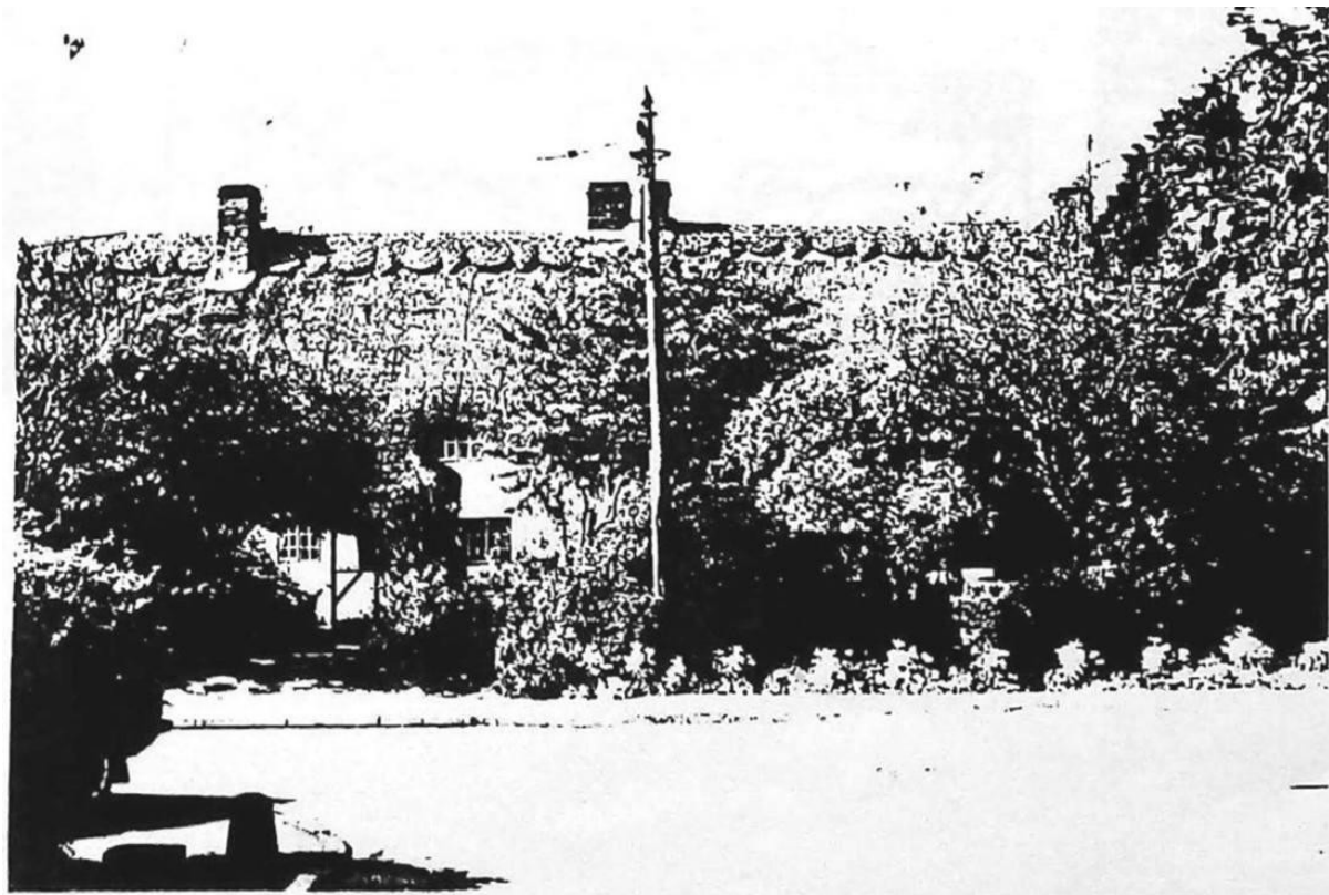
Nos 1 to 3 Chapel Street and Cleve Cottage, "a range of four cottages, C17, timber framed faced in plaster, continuous thatched roof, one storey and attic" (Conservation Area Study, July 1992, Building Ref 26; 15/08, p.4).
